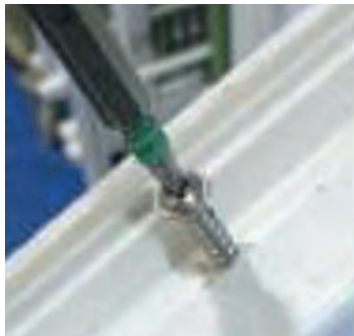
Loosen screws on the side of the sash but do not remove.
