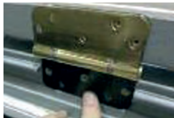
Fixed pin hinge shown locating into pre-formed cut out.
